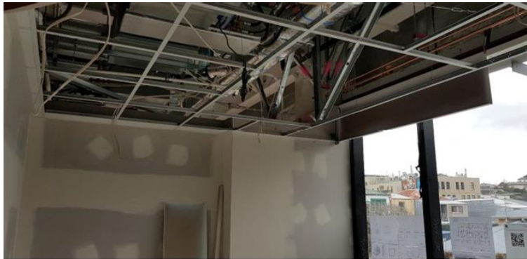
Level 2 ceiling framing & wall linings
