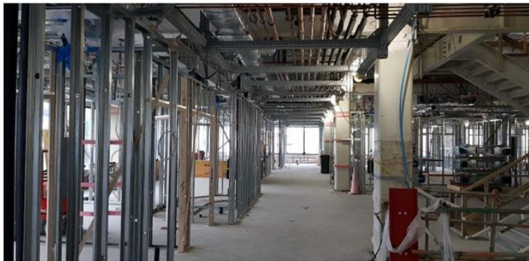
Level 3 wall framing and services first fix
