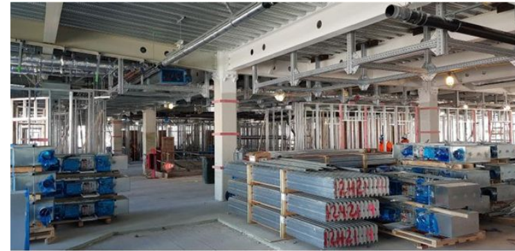
Level 4 – Bedroom wall framing & Services 1 st Fix
