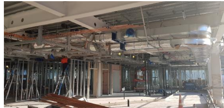
Level 3 wall framing and services first fix
