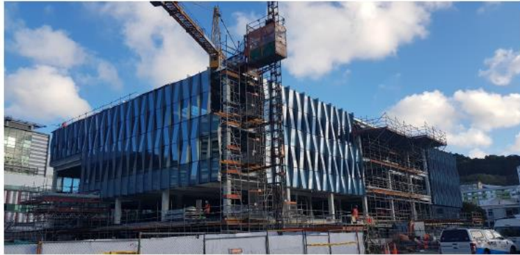
Exterior North & East Elevations
