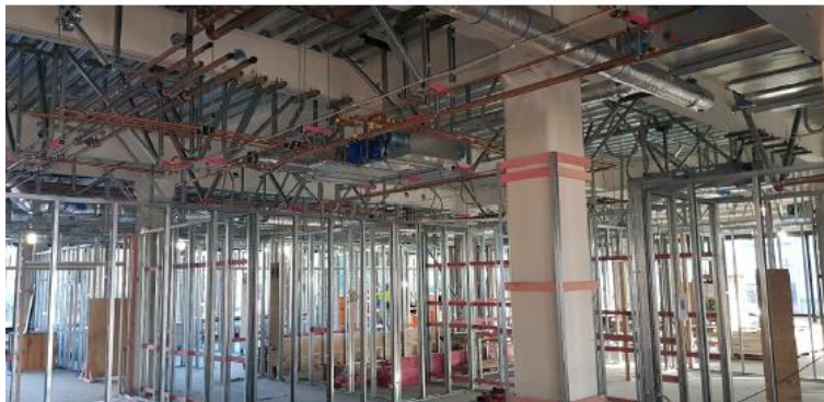
Level 2 wall framing and services first fix
