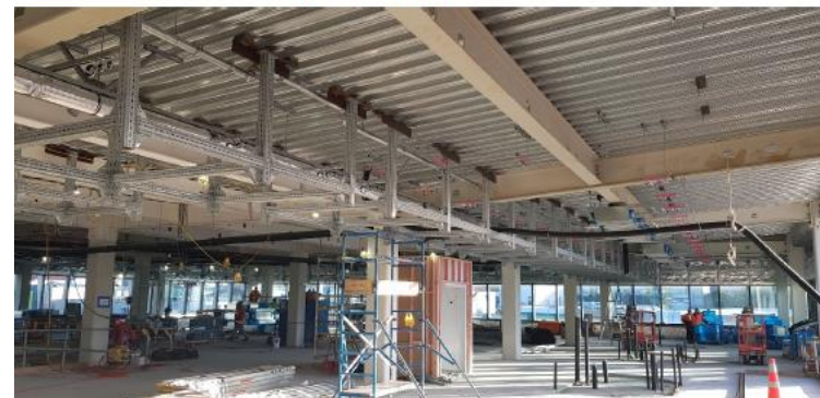
Level 4 wall framing and services first fix
