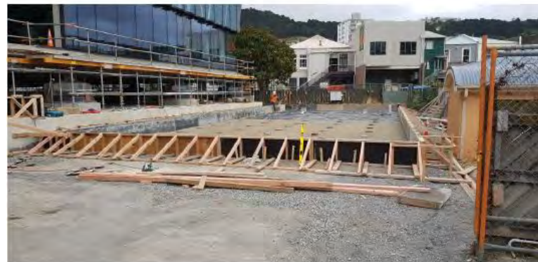
Services Annex Raft Formwork
