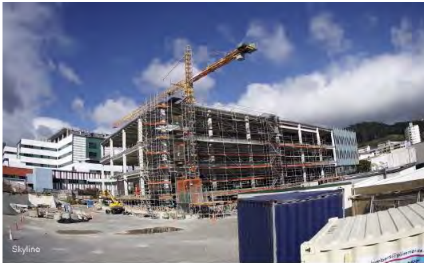
Exterior North & East Elevations
